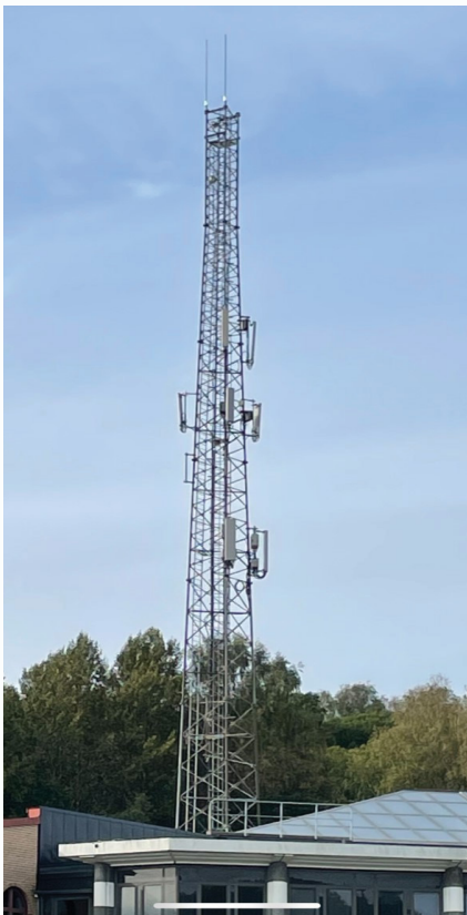
Figure 1: Mast with 5G base stations 200 meters from the school.
